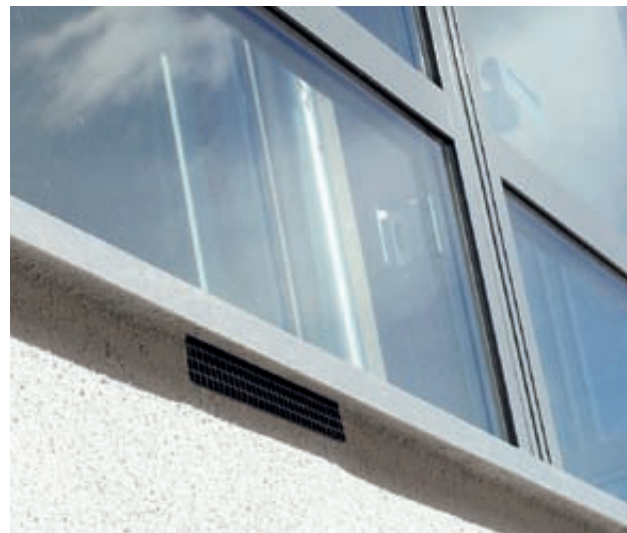
An example of concealed air intake below the window ledge flashing
